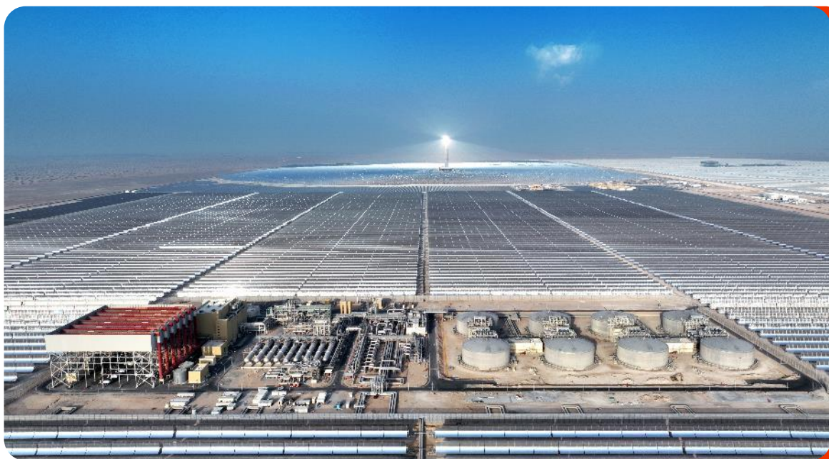
Mohammed bin Rashid Al Maktoum Solar Park
